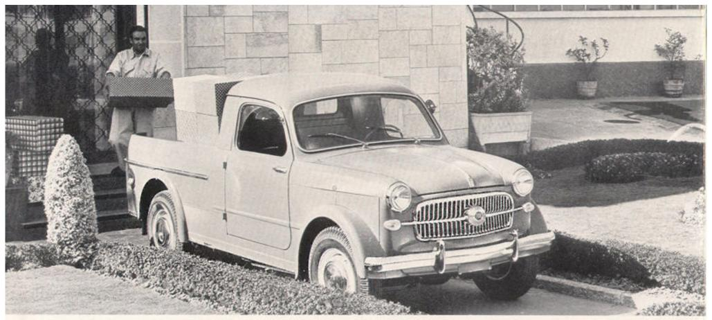
Enclosed cab, side panels in one piece with side panelling of body, all-metal construction with stressed internal framework. Two doors. Back of cab provided with large centre window of safety glass with protective metal bars. Two seats. Box body with fixed sides and drop tailboard.
